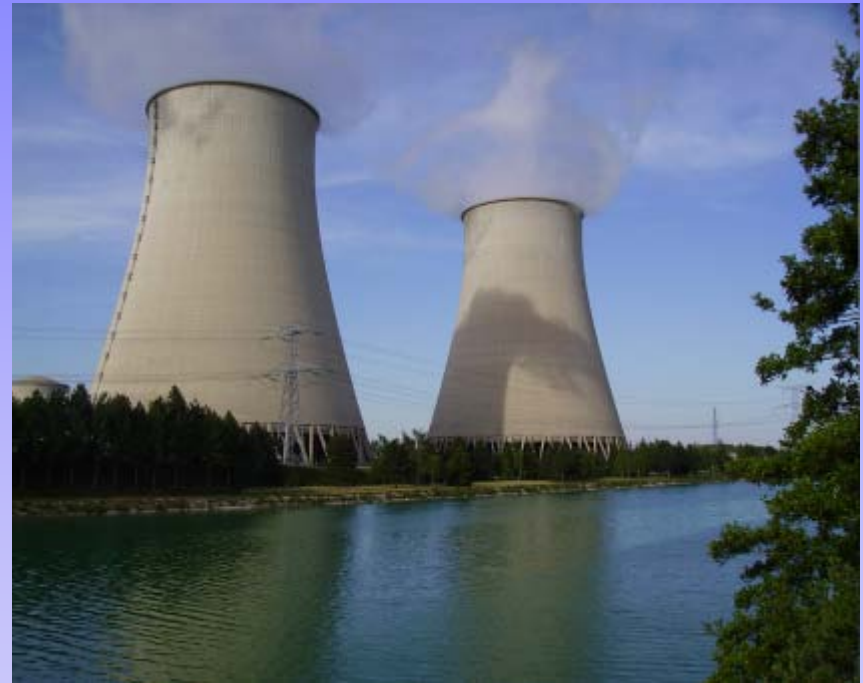
France Nogent Nuclear Power Plant ZETA 2 x 24MW, 6.6kV, 15 bar Aux Boilers
